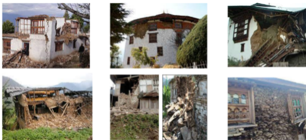
Figure 1: Past earthquake damages on traditional Bhutanese structures
