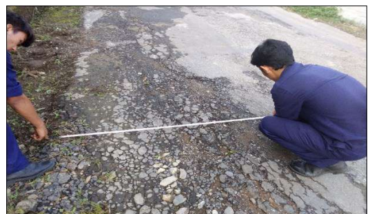
Fig. 5. Alligator Crack
